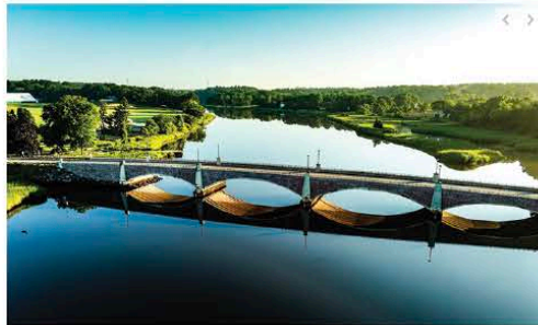
"Berkley Bridge Reflections" by William Gibson; photography
